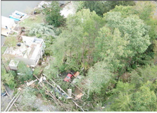
Tornado Damage – Lake Lanier, SC 2017
