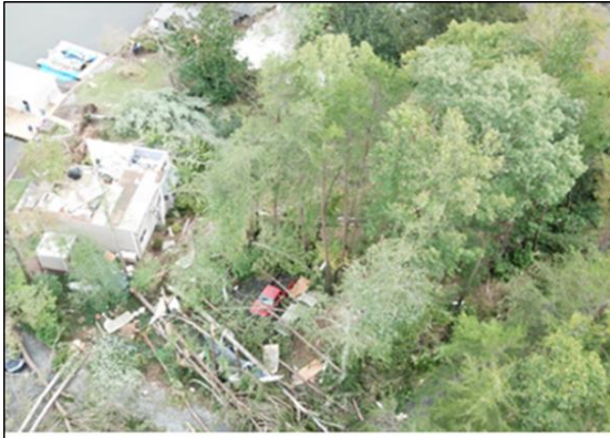
Tornado Damage – Lake Lanier, SC 2017
